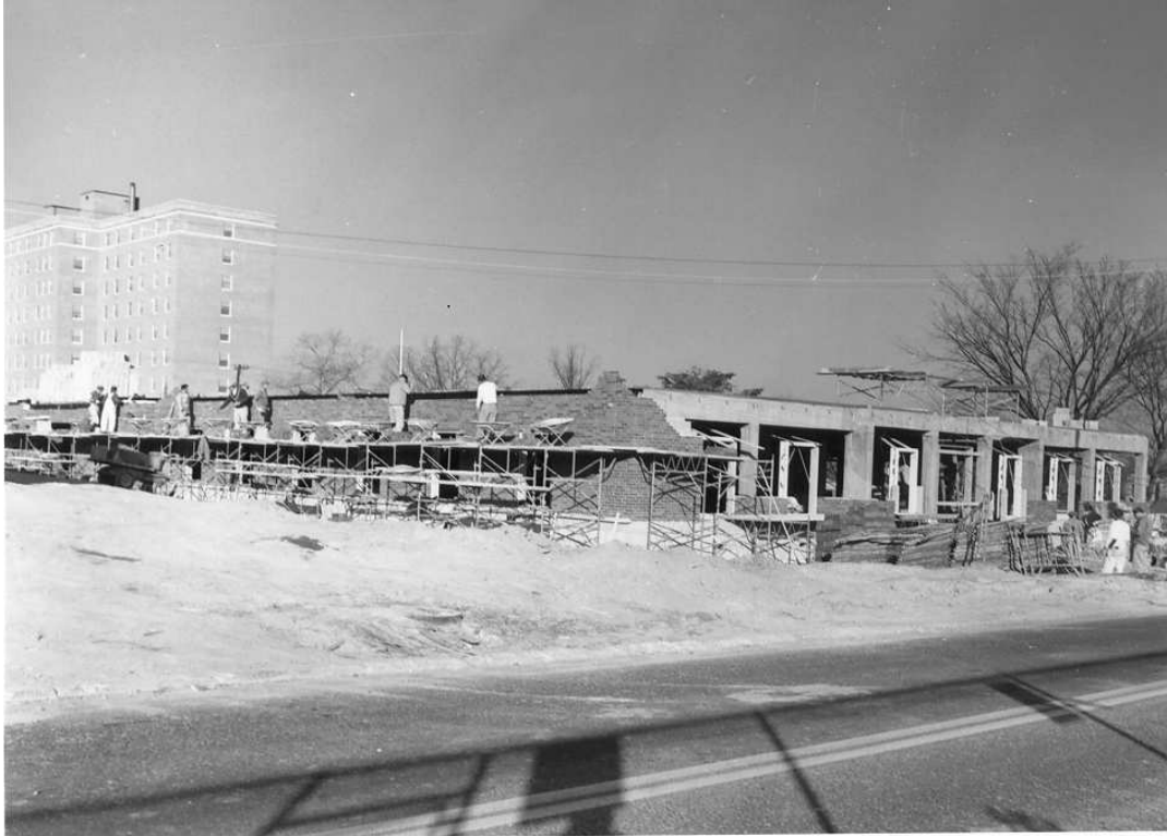
Figure 3: Computer Science Center Building, November 1962, Completion of Bricking-in of First Floor, Centerville Hall in background, Courtesy of John Menard.
